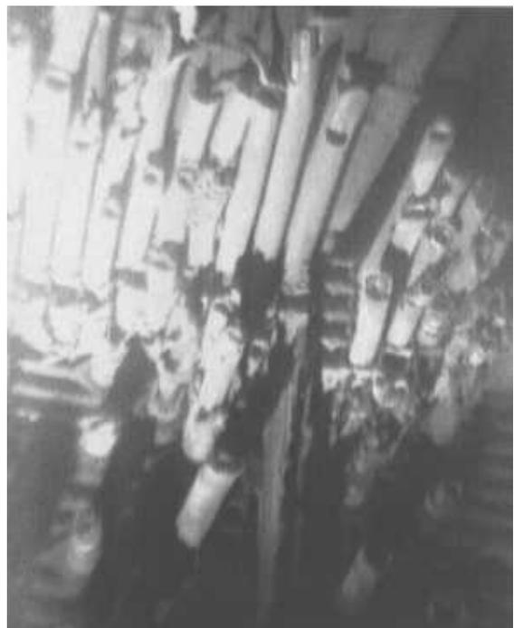
for vessel confirmed the existence of another bed of rubble at the bottom of [lie reactor.
