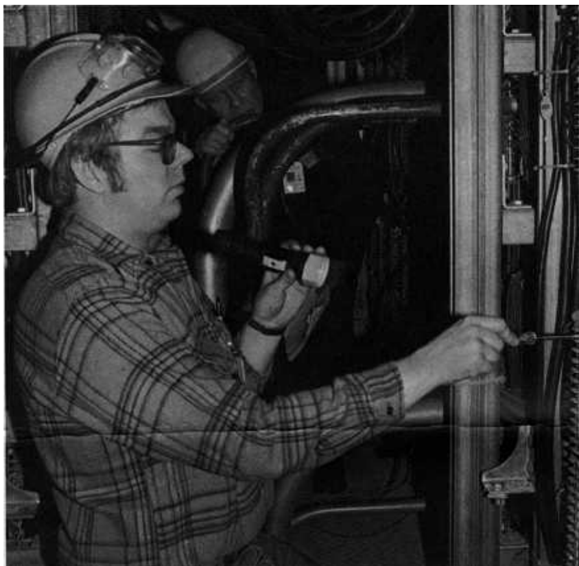
Electricians check circuits beneath the Unit 1 control room. As part of the Unit 1 restart program, all electric circuits in the unit are being checked to ensure safety and readiness for return to service.
