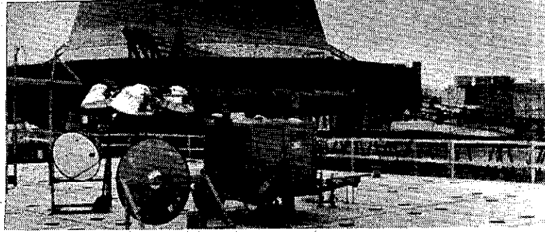
A TMI cooling tower is quiet now.
